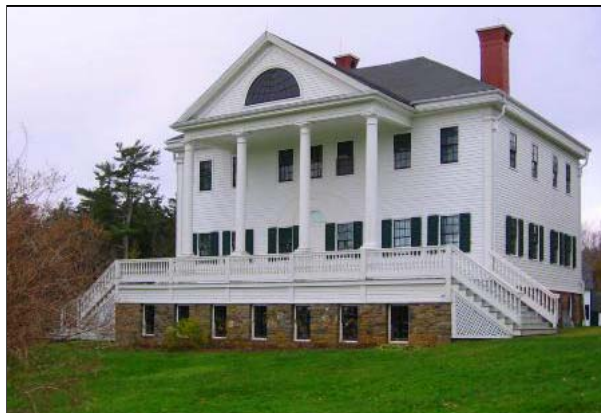
Canada needs stable entry-level housing for its homeless singles population. Traditionally this has been provided not by the government but by the private sector single room occupancy unit (SRO`s) in rooming houses, older hotels, and smaller apartments.
